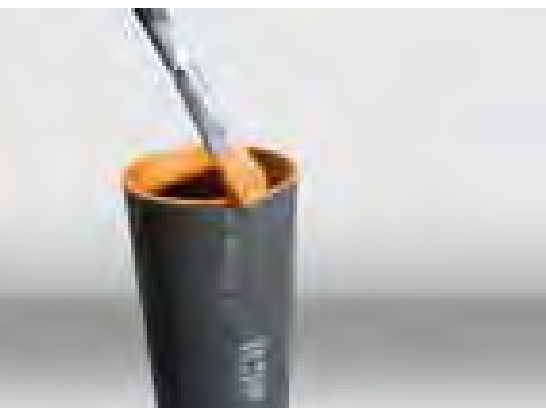
An edge seal coating should be applied to the cut edges before they are joined together. This can be sprayed on or applied with a brush (DIN EN 1610 8.5.5)
